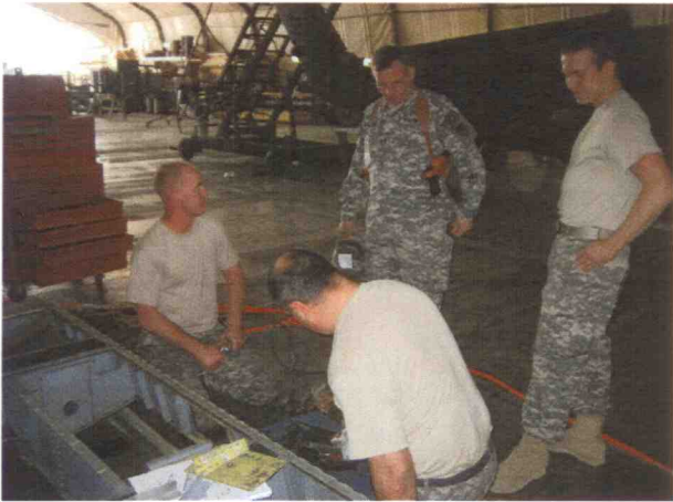
CW2 Mike “Grayfox” Gray advises SSG Rick Consdorf, SGT Jonathan Malone, and SPC Robert Johnson on the procedures for a structural repair on the CH-47 Chinook ramp.
